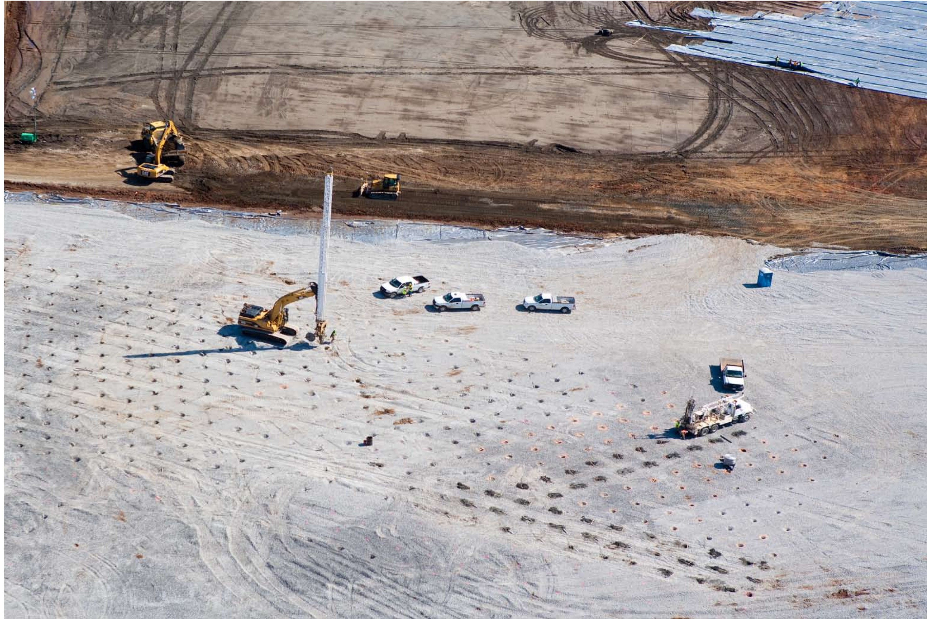
Placing the wick drains
