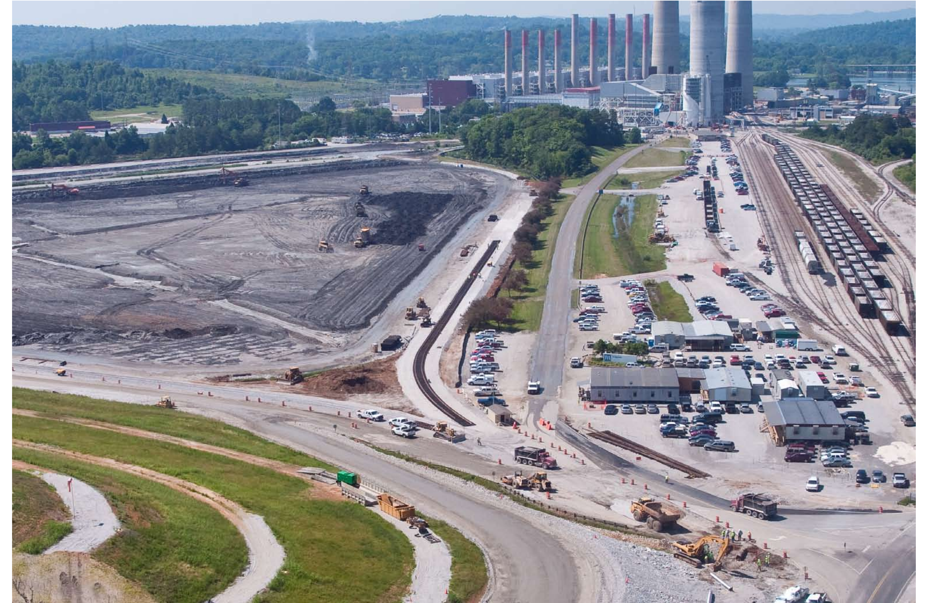
Railroad spur construction
