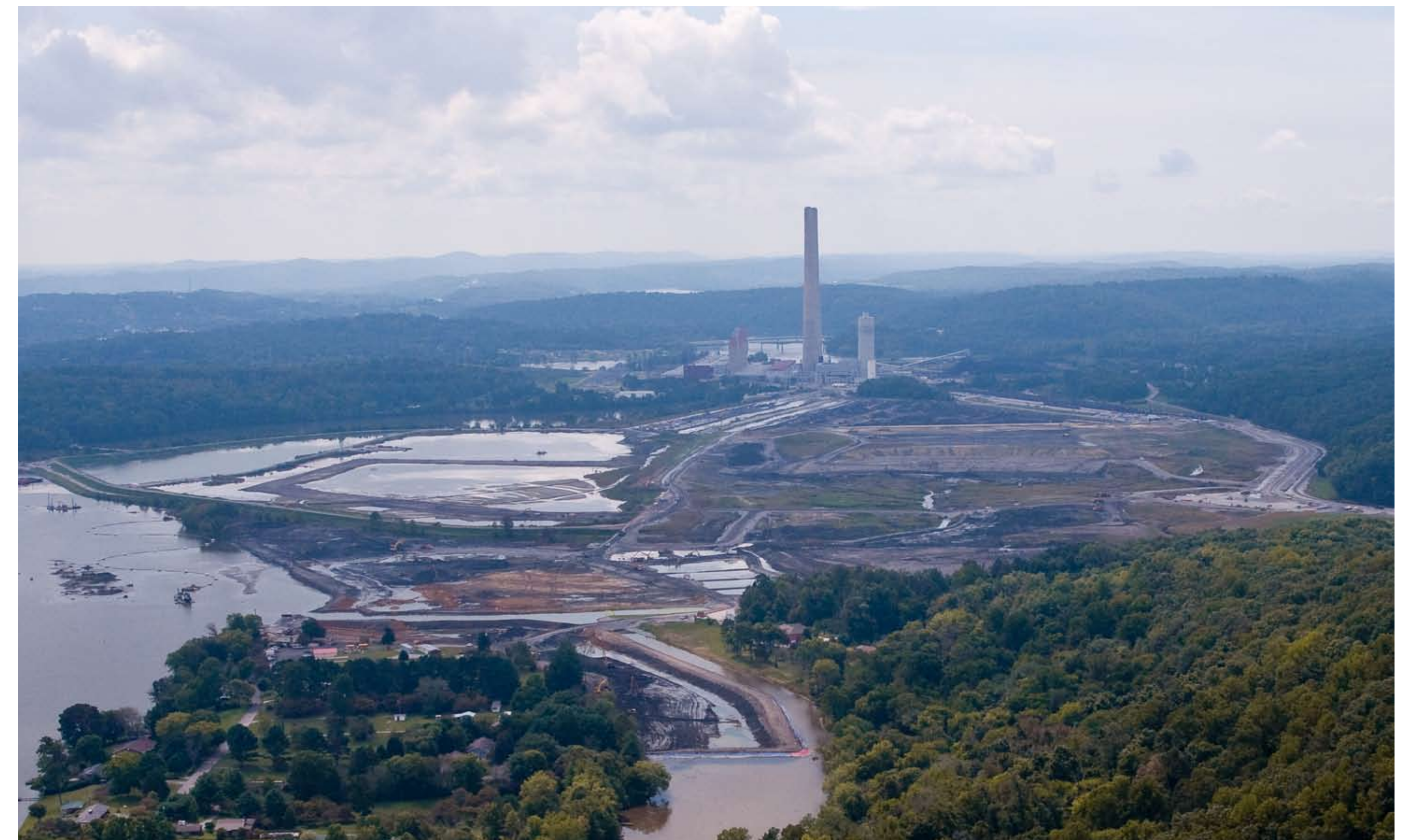
Dredge cell before and after
