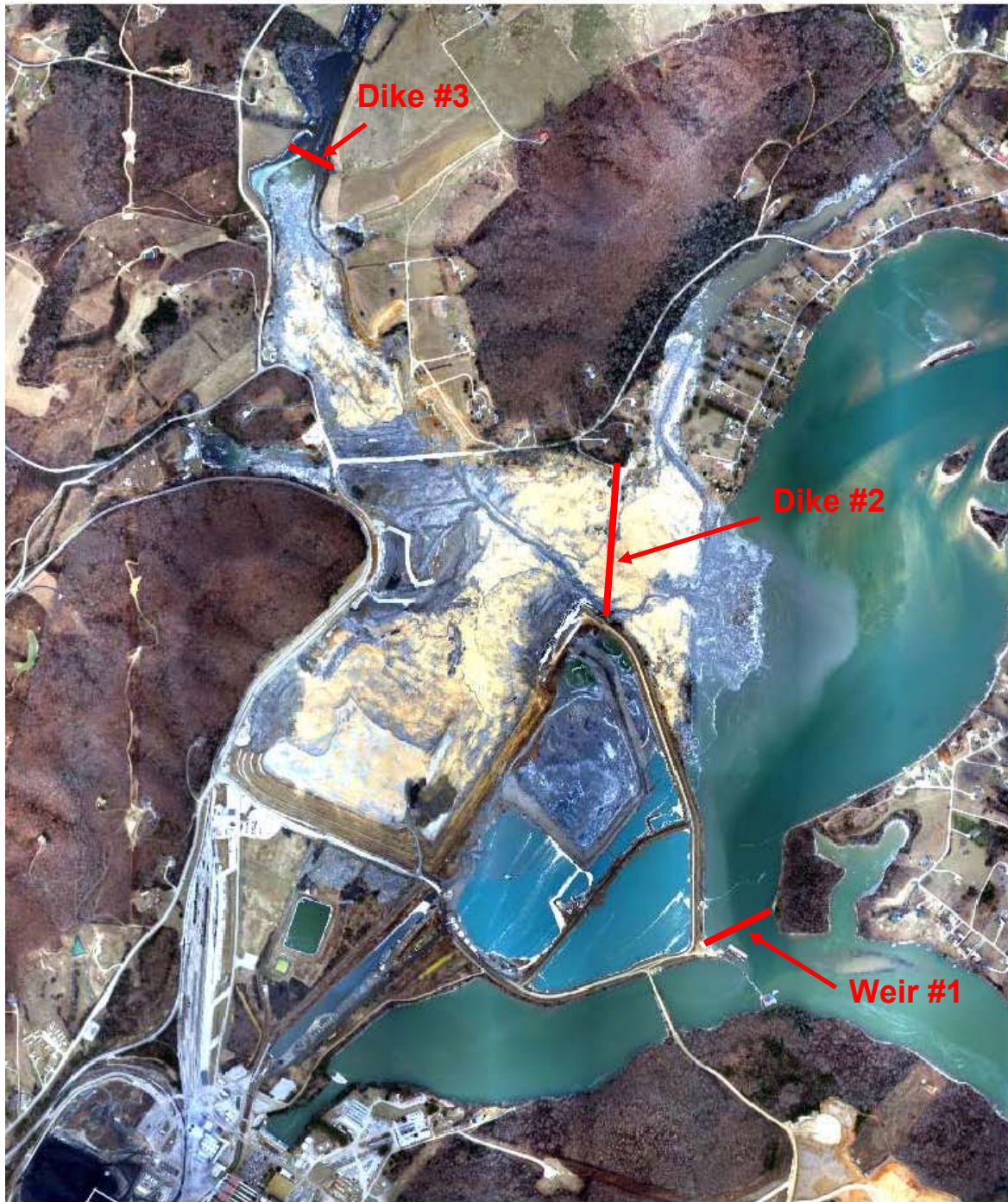
Aerial Image of Kingston Ash Slide 01/17/2009
